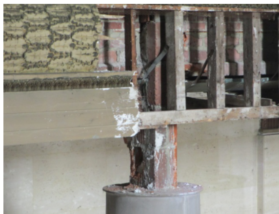
Figure 49. Exposed Top of Steel Clerestory Column
