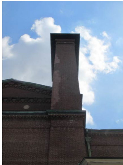
Figure 33. Northwest Flue Stack Brick Replacement
