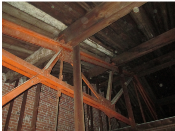
Figure 15. Steel Roof Truss Supporting Heavy Timber Framing
