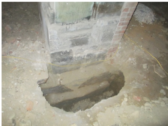
Figure 56. Stone Foundations Beneath Clerestory Columns
