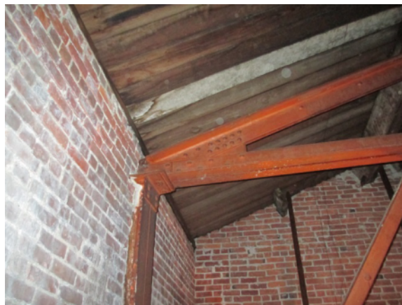
Figure 17. Steel Plate Girder Column Embedded in Wall
