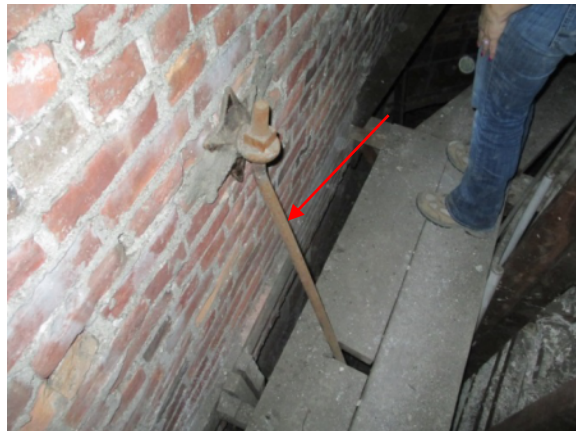
Figure 10. Steel Hangers at Interior of Drum
