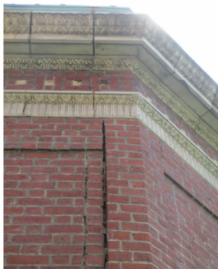
Figure 46. Close-up of Brick Separation at Northeast Elevation
