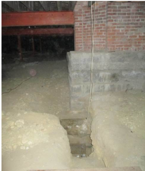
Figure 54. Stone Foundation for Interior Brick Pier
