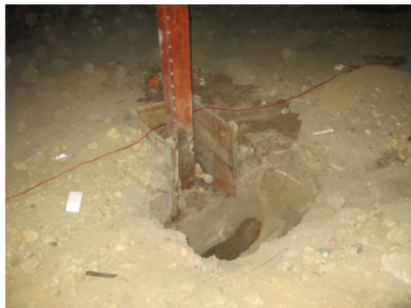
Figure 57. Concrete Spread Footing Interior Steel Columns
