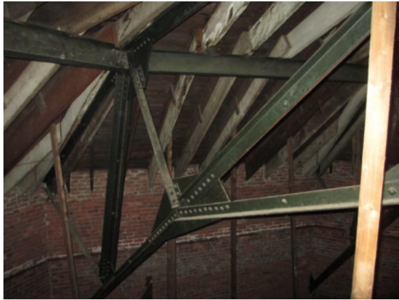
Figure 7. Radial Steel Trusses
