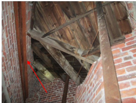
Figure 12. Steel Channel at Exterior of Drum for Hangers
