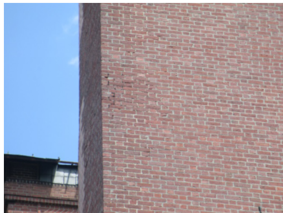
Figure 31. Northeast Flue Stack Brick Damage (Close-up)
