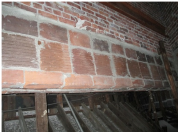
Figure 9. Terra Cotta Encased Steel Beam at Base of Drum
