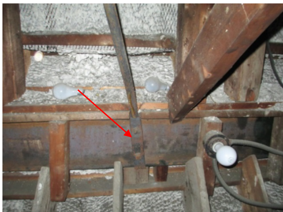
Figure 11. Steel Hanger Picking Up Steel Channel "Ring"
