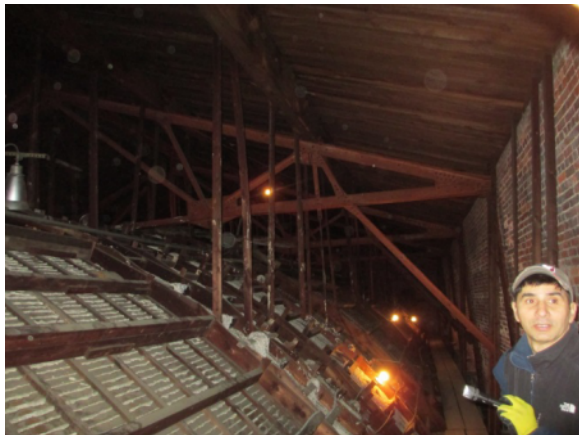
Figure 14. Steel Roof Truss
