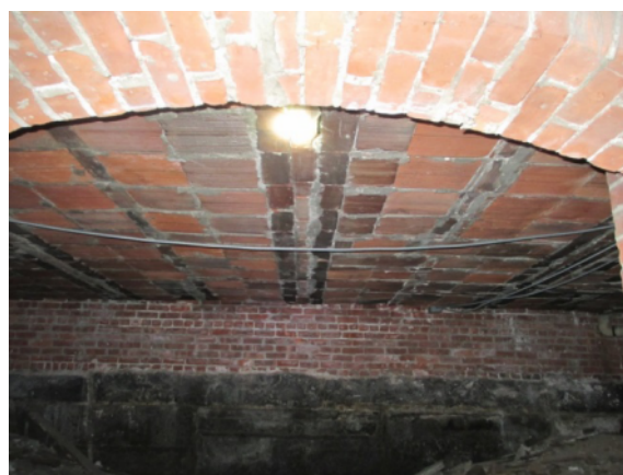
Figure 53. View of First Floor Structure Beneath Narthex
