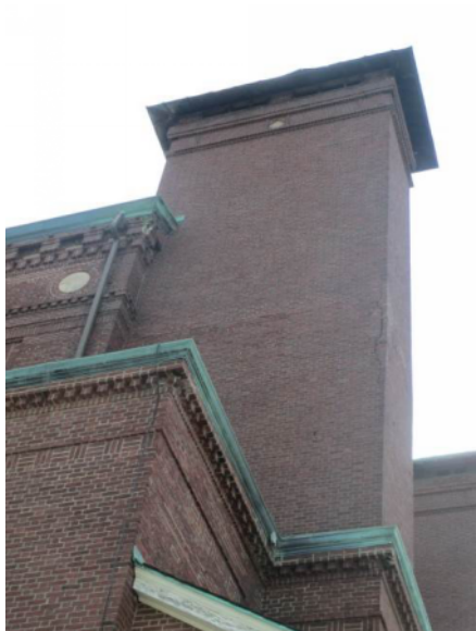
Figure 32. East Elevation of Northeast Flue Stack Showing Brick Bulging Out of Plane
