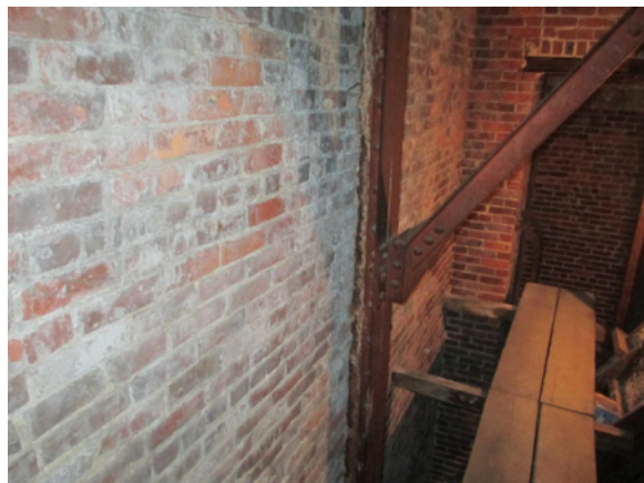
Figure 16. Steel Plate Girder Column Embedded in Wall
