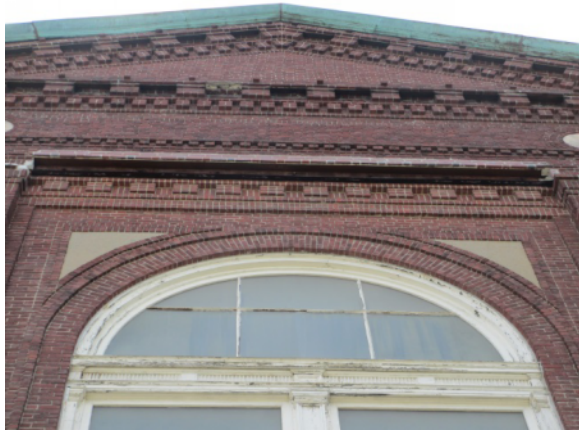
Figure 26. East Transept Steel Lintel with Missing Brick
