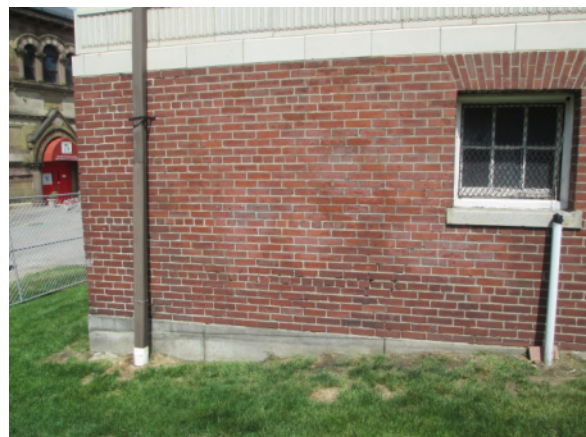
Figure 43. Northwest Corner With Minor Step Cracking
