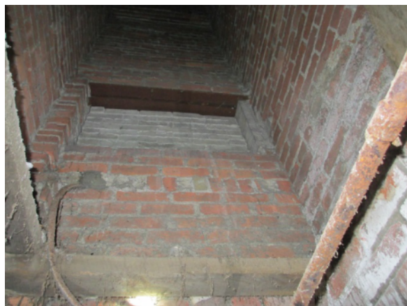
Figure 35. Previous Opening in Flue Stack Blocked Up
