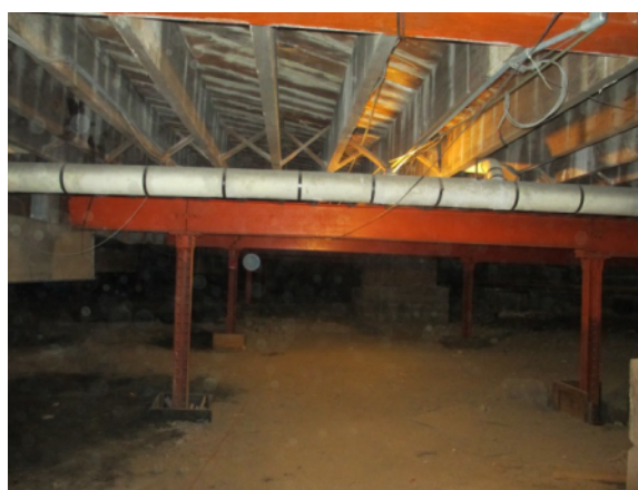
Figure 51. Underside of First Floor Framing from the Basement
