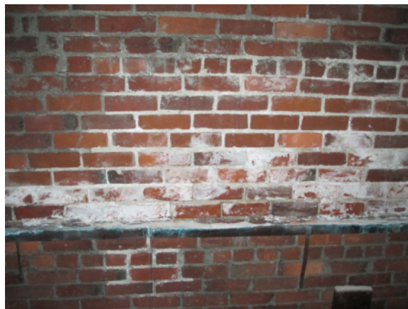
Figure 21. Efflorescence at Interior of Drum
