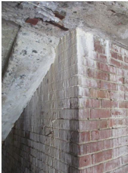
Figure 40. Efflorescence Deposition on Building Wall
