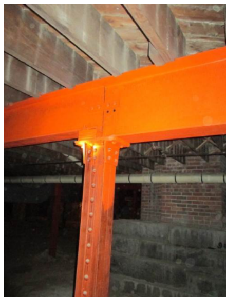
Figure 52. First Floor Interior Steel Beams and Column
