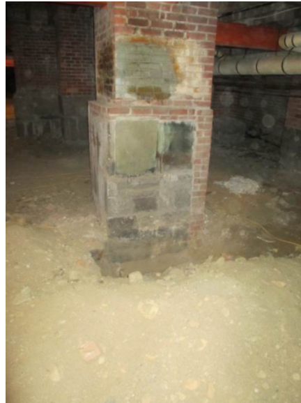
Figure 55. Brick Pier at Clerestory Column Footings
