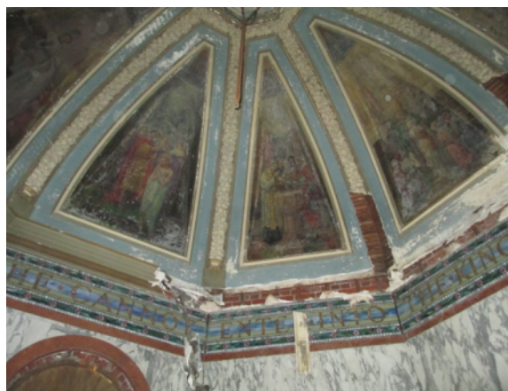
Figure 47. Plaster Damage on the Interior of the Baptistry
